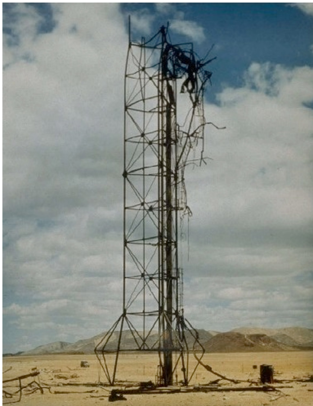
Figure 25. Post-test remains of the Ruth event test tower.
