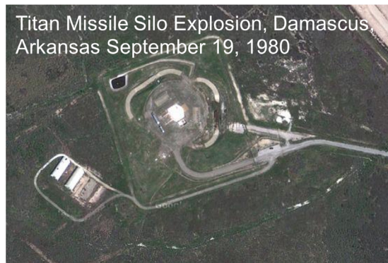
Figure 33. Aerial view of Titan missile silo installation (U.S. Air Force photo).
